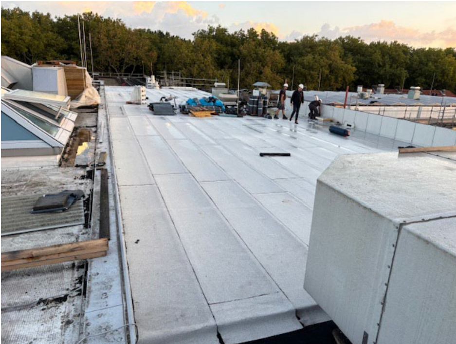
Dak 20-gang is gereed.
